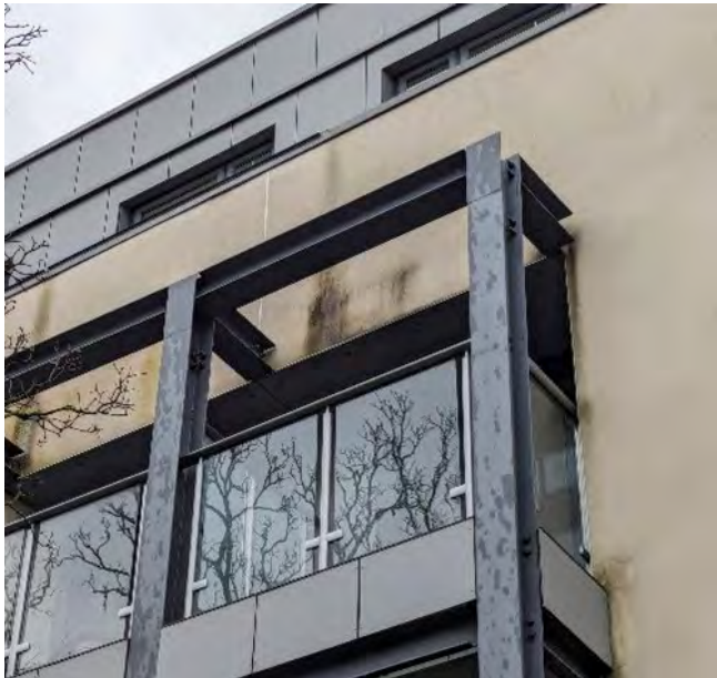
New build apartments in West Bridgford. A combination of the interface of steel balconies, mechanical ventilation extract/ intake and pollution with light coloured renders result in staining/discolouring.
